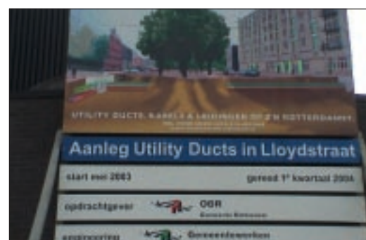
Foto 4. Utility ducts in Rotterdam (foto Jan Prins).
